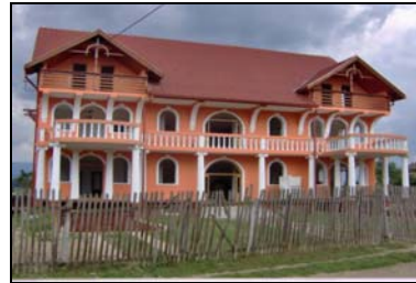
Photo 4. Boarding house under construction. 1
