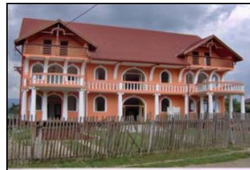
Photo 4. Boarding house under construction. 1
